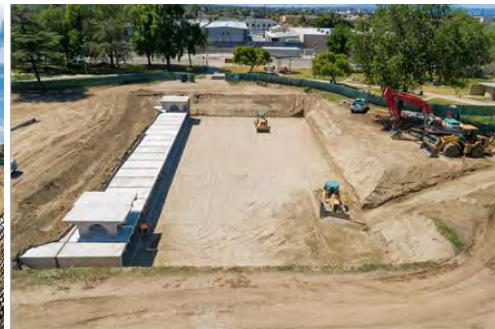
Underground Storage – Carriage Crest Park Diversion Project in Construction (Moon and Passanisi 2020)
