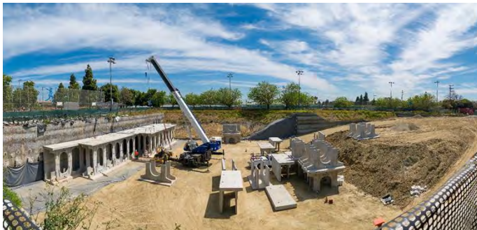
Underground Storage – Carriage Crest Park Diversion Project in Construction (Moon and Passanisi 2020)
