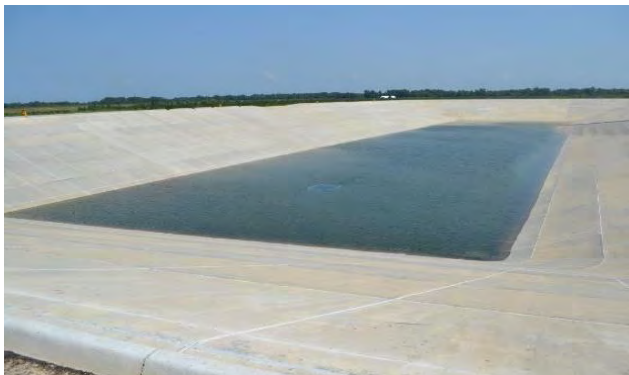
Belowgrade Open Earthen Basin
