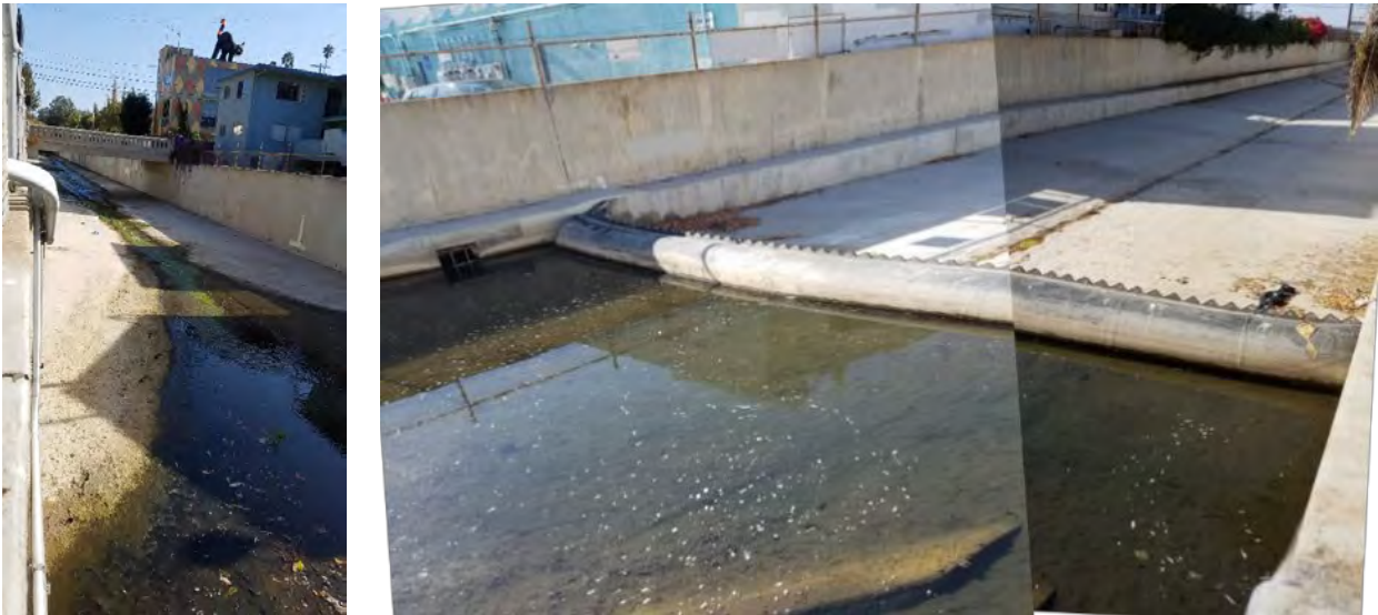
(a) Upstream of Diversion (b) Diversion Dam and Downstream
